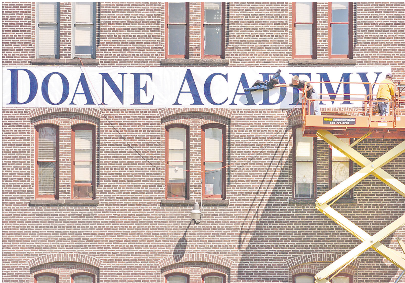
Joe Seib (left), and Chuck Magee maintenance workers at the school previously known as St. Mary's Hall-Doane Academy, hang a banner announcing the renaming of the 171-year-old school in Burlington City. The school is now known as Doane Academy. BCT staff photo/DENNIS McDONALD
